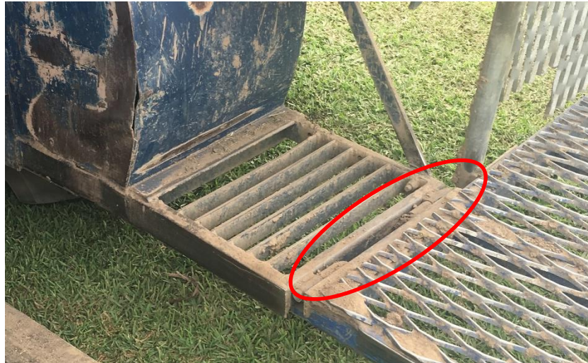
Figure 10 Hinge Area of Concern
