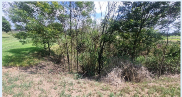
Dense brush, woody trees (This drain is in poor condition and might be blocked by trees and woody debris)
