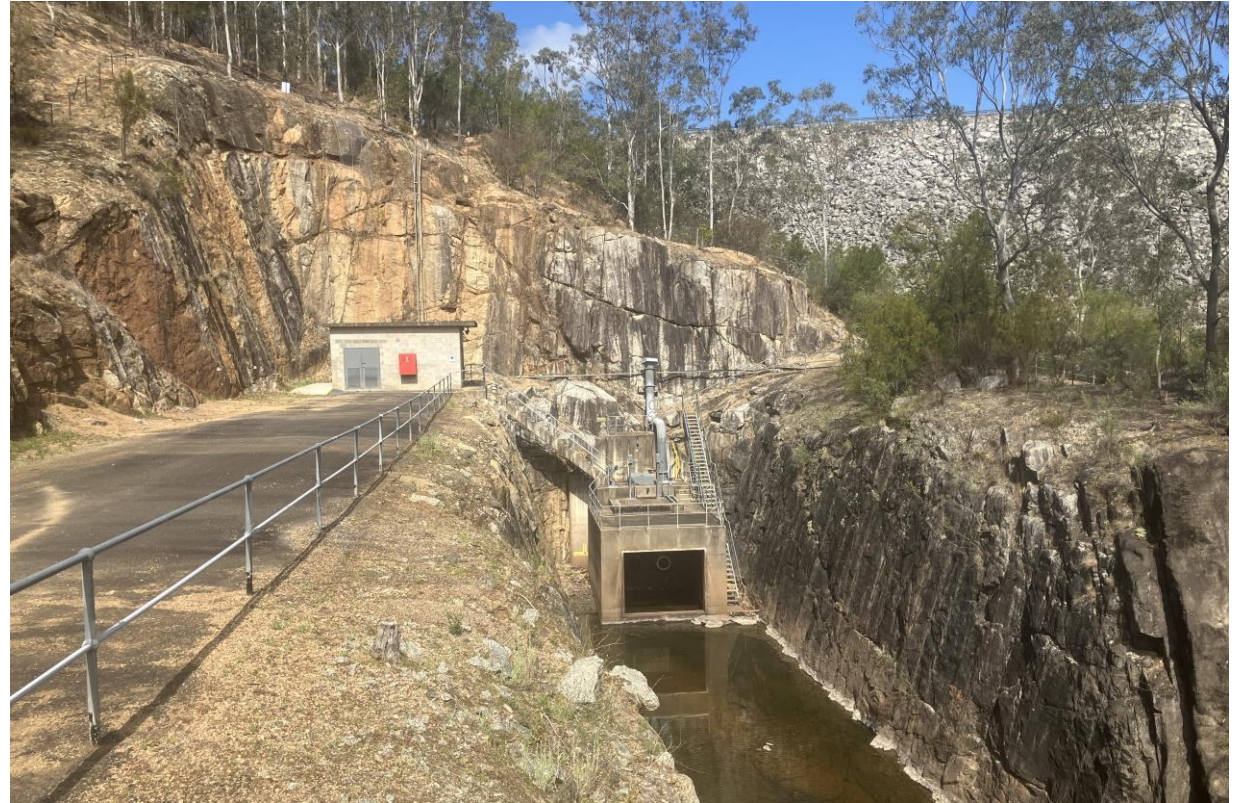
Brogo Dam valve house
